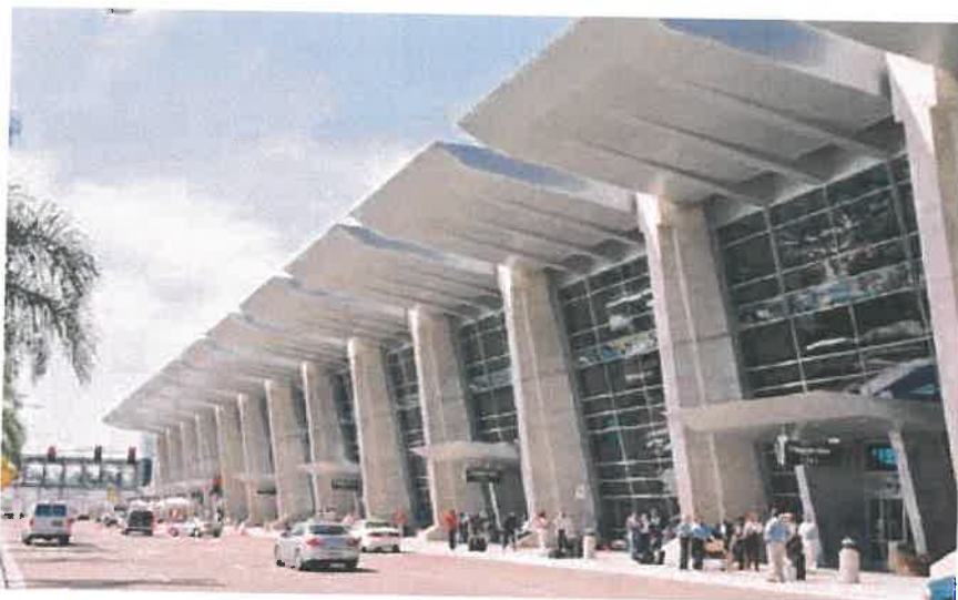
Rehabilitation of Terminal 2 West, Lindberg Field San Diego
