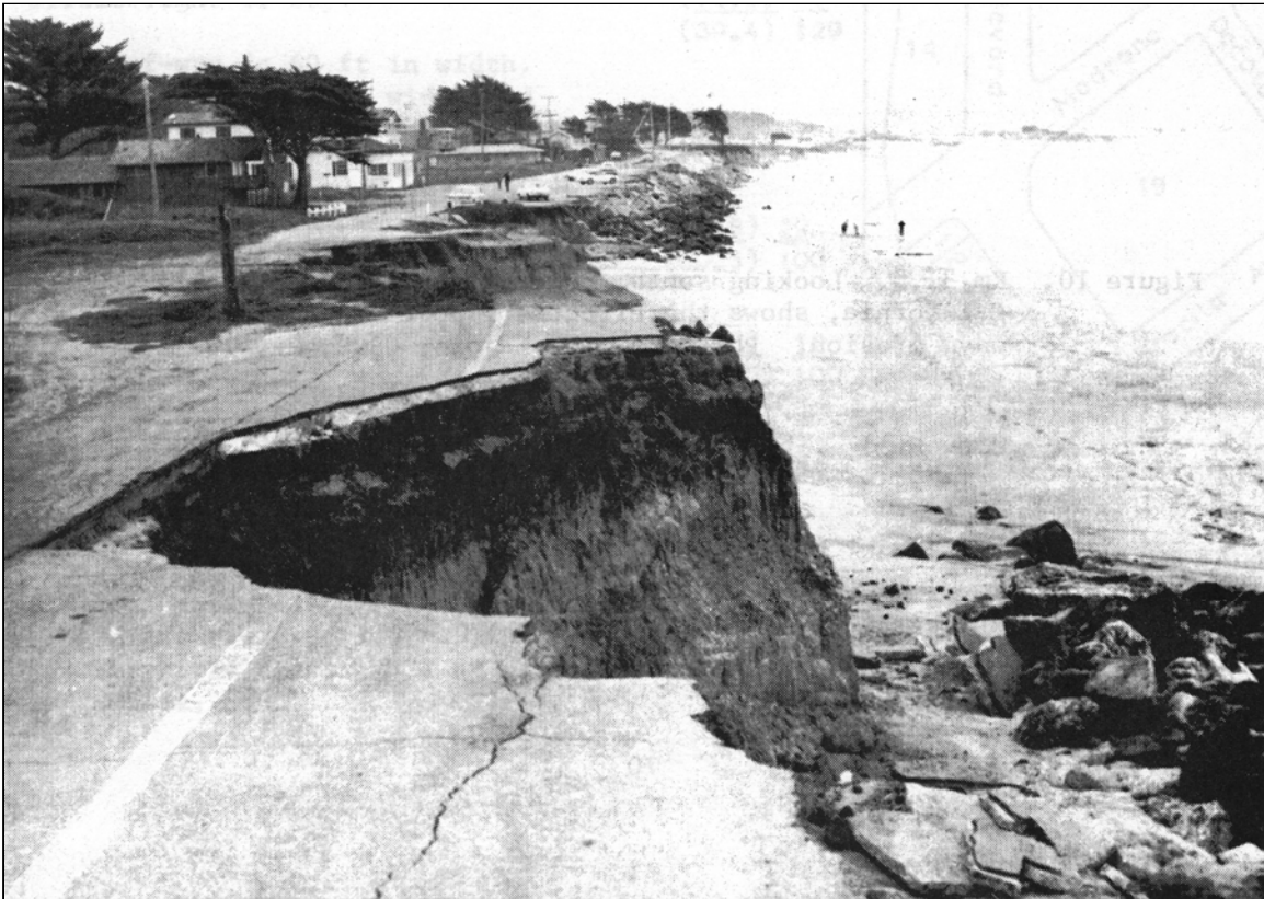
Figure 7: 1971 photograph of Mirada Road looking south from near the root of the East Breakwater. Subsequently, the road was destroyed. Rip-rap can be seen along the sea cliff starting at about the white house and going south. Photograph by K. Lajoie, USGS.
