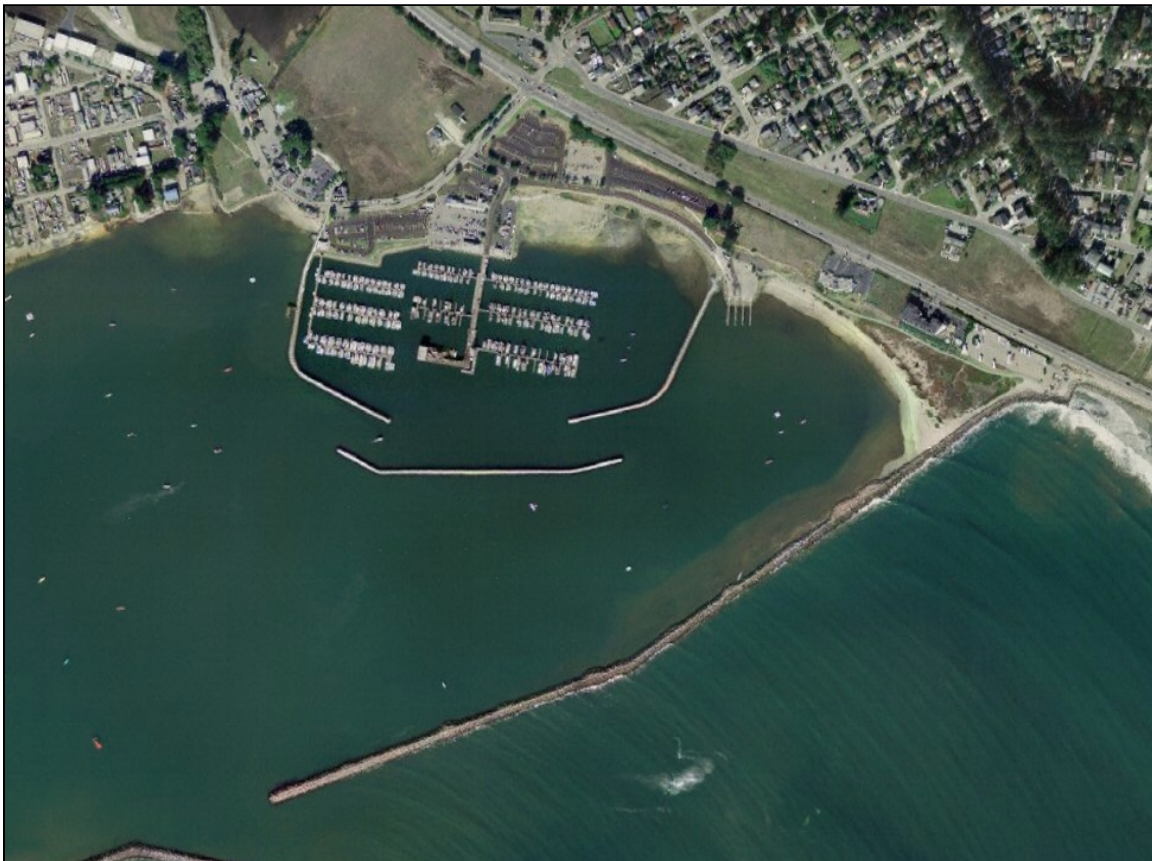
Figure 5: East end of Pillar Point Harbor showing East Breakwater, inner breakwaters, and inner beach adjacent to the root of the East Breakwater.
