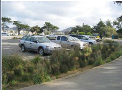
Bioswale Storm Water Treatment (Mix of sedges and rushes adjacent to marina parking area)
