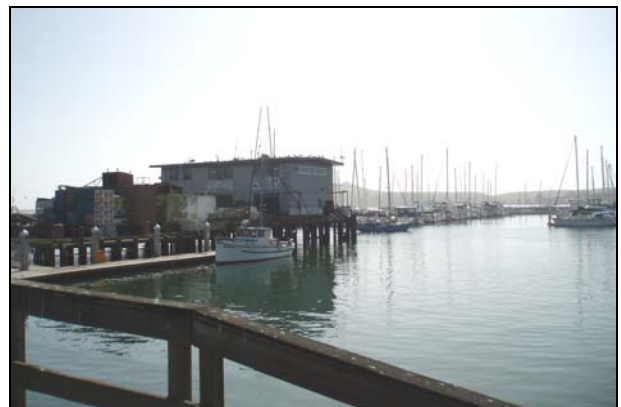
Figure 47: The facilities found at the end of Johnson's Pier in Pillar Point house three wholesale fish buyers. Photo by Barbara Stickel, May 2, 2006.
